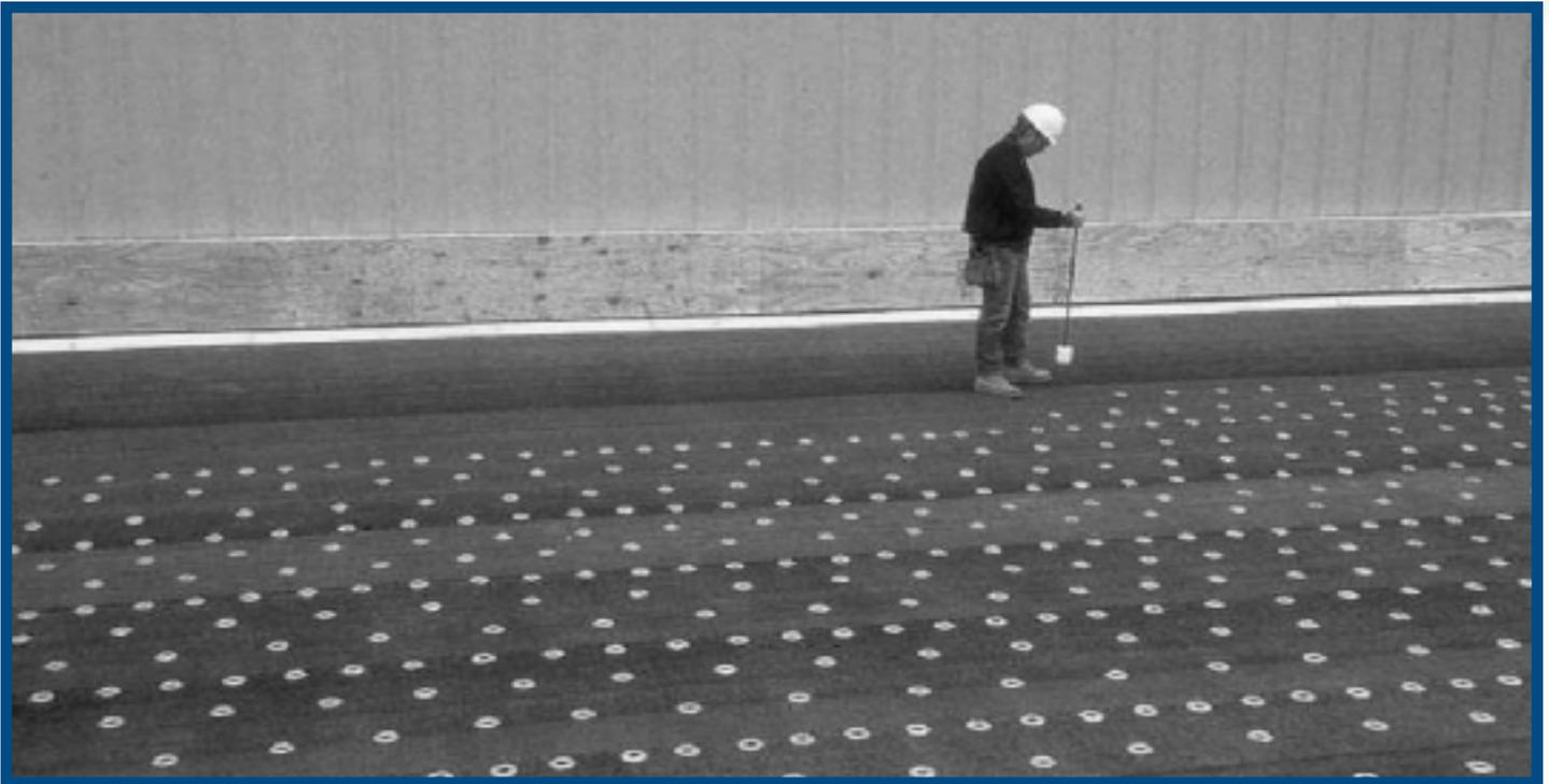
*Nailing the base sheet to a lightweight insulating concrete deck.*
