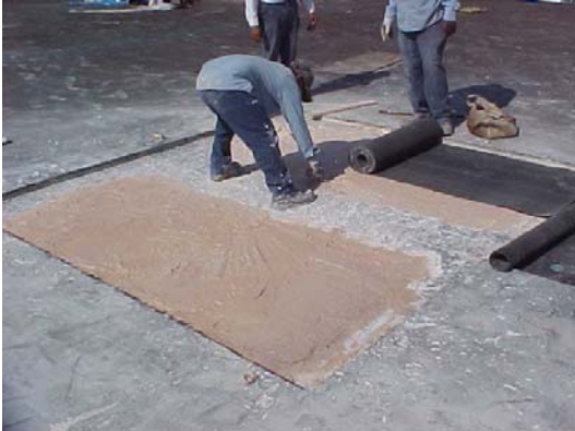
13. Rolling Out New Base Sheet
