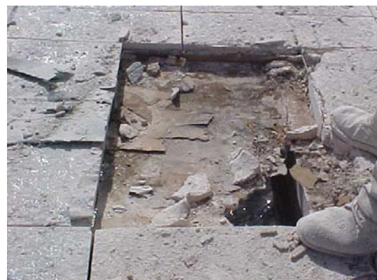
5. Cutting Section from Deck
