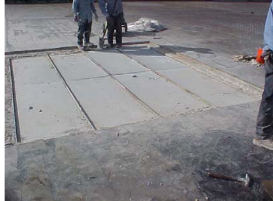
9. Complete Installation of New Form Board
