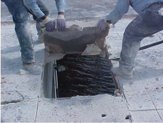
6. Removing Cut Section
