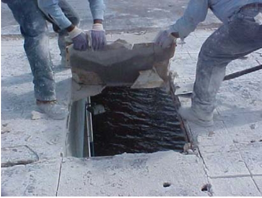
6. Removing Cut Section
