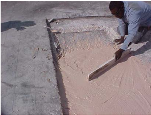
12. Installing New Gypsum Concrete and Smoothing Surface
