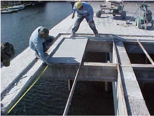
8. Installing New Form Board in Repair Area
