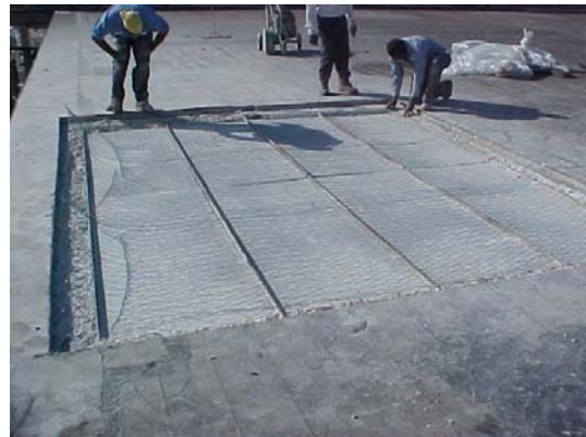
11. Completed Installation of New Wire Mesh
