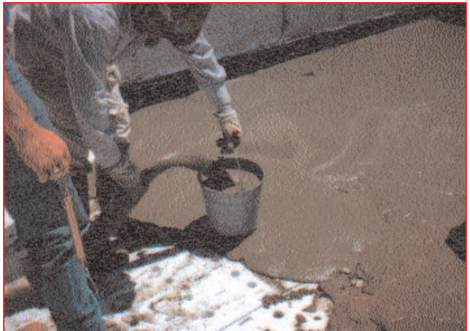
Photo 1: A 10-quart steel pail is commonly used for the "pail test."
